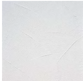
Stucco (outer wall)
